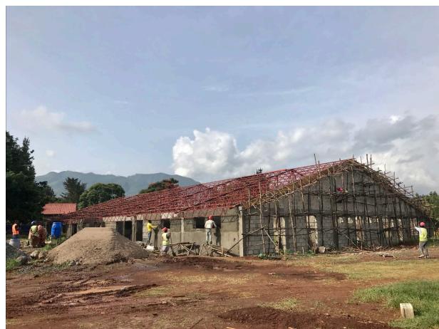
The new surgical suites are also making good progress.
